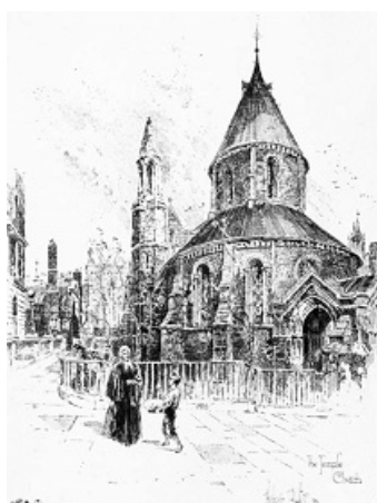
The cupola was added later by Smirke and no longer exists
