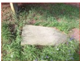
Before being re-erected on new base
